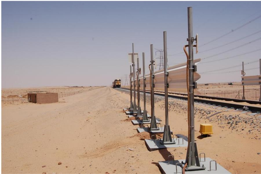
Sensor data from temperature and weight sensors are combined with RFID read events thus providing complete train lists with trailer numbers for safety checking. The solution is especially build for the hot and dry climate of the Saudi Arabian dessert with temperatures up to 50° Celsius and resist winds with up to 200 km/h.
